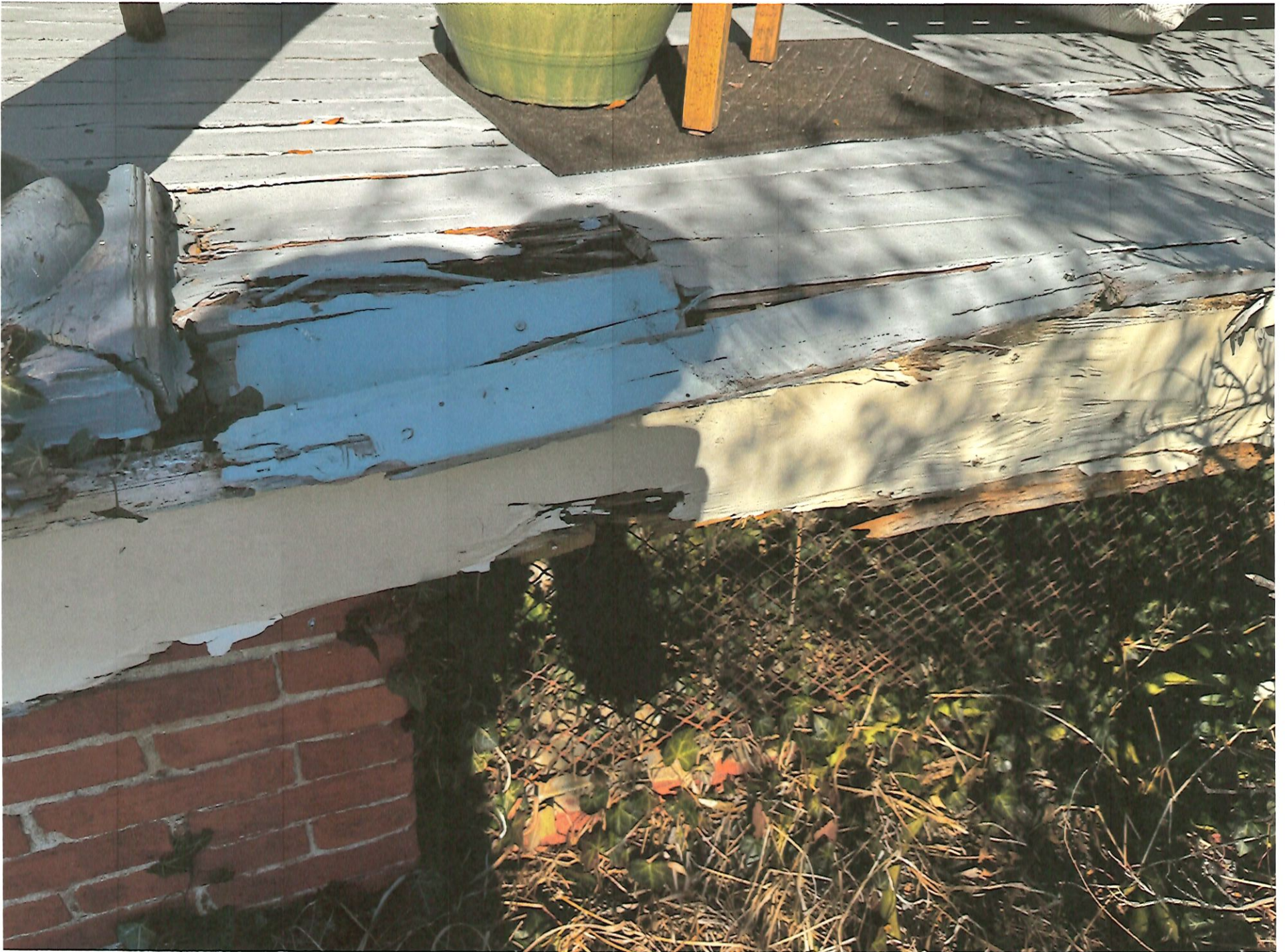
Front porch - south side
